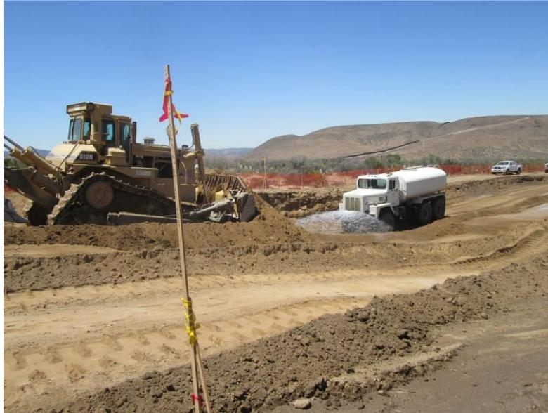
**Photo 1:** Water trucks are utilized during grading activities to minimize fugitive dust in accordance with Mitigation Measure BIO-4a and the Dust Control Plan.
