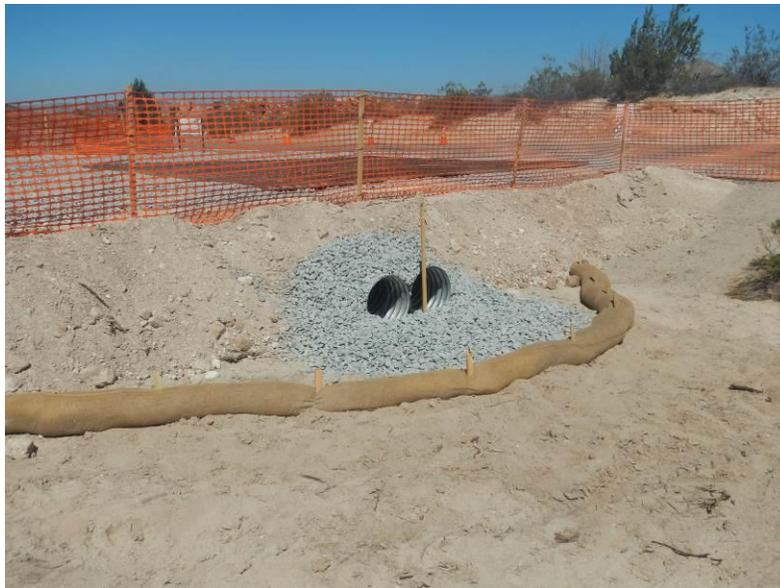
**Photo 2:** BMPs are installed along the right-of-way to minimize the potential for erosion in accordance with Mitigation Measure HYD-1 and the SWPPP.
