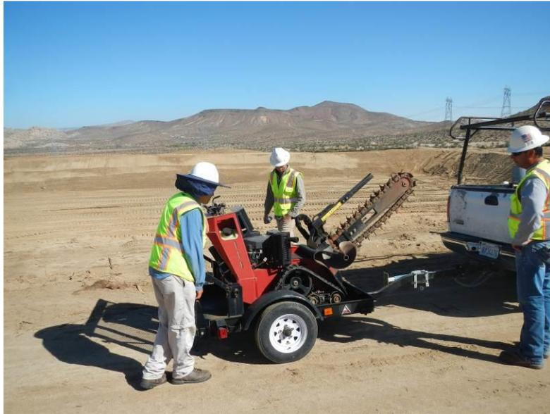
**Photo 5:** Construction equipment is inspected and verified to be clean and free from dirt and debris prior to being unloaded on-site to minimize the spread of invasive plant species in accordance with Mitigation Measure BIO-3a.
