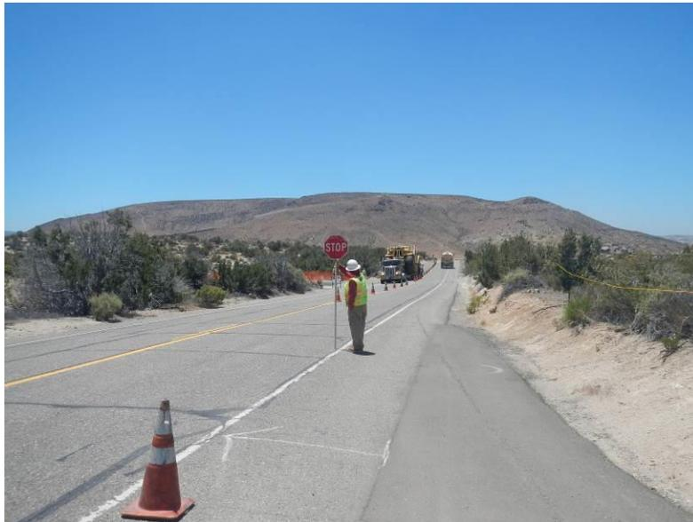
**Photo 4:** Traffic cones and flaggers present along Old Highway 80 in accordance with Mitigation Measure TRA-1.
